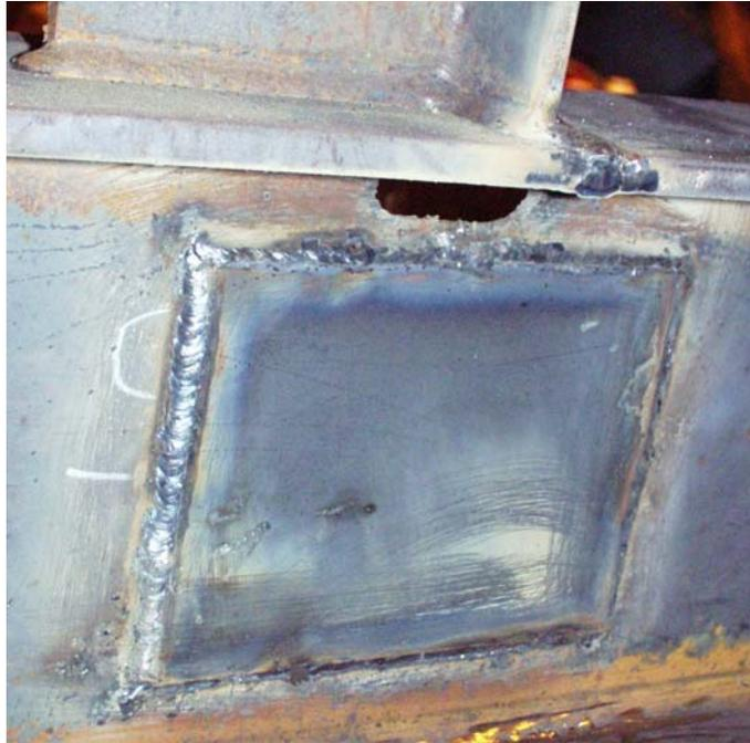
Figure 22: Welded doubler plate
