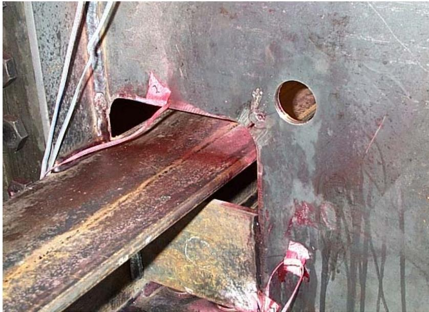
Figure 3.49 Typical stop hole repair in web frame
