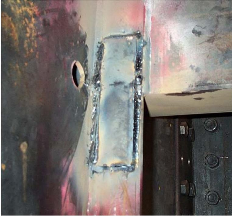
Figure 3.88: Doubler welded to flat bar stiffener (specimen 2)
