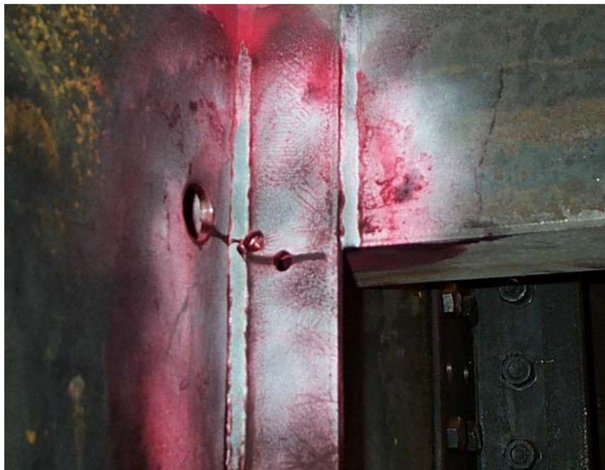
Figure 3.87: Ineffective 14 mm stop holes in flat bar stiffener (specimen 2)
