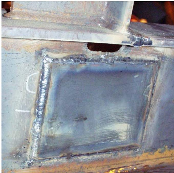
b) Repair of crack.
