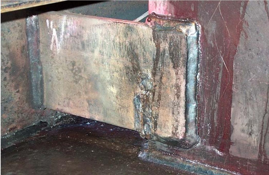
Figure 3.59 Weld repair in cracked lug plate (original crack shown in Fig. 3.54)
