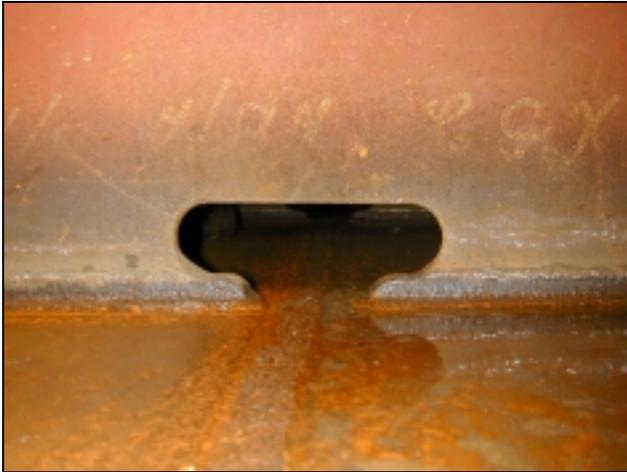
**Fig. A4** Typical “Mushroom” Cutout at Erection Joint in Ballast Tanks
