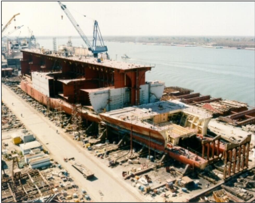
**Fig. A8** Photo from Stern Looking Forward (Note Twin Skeg Arrangement Aft)
