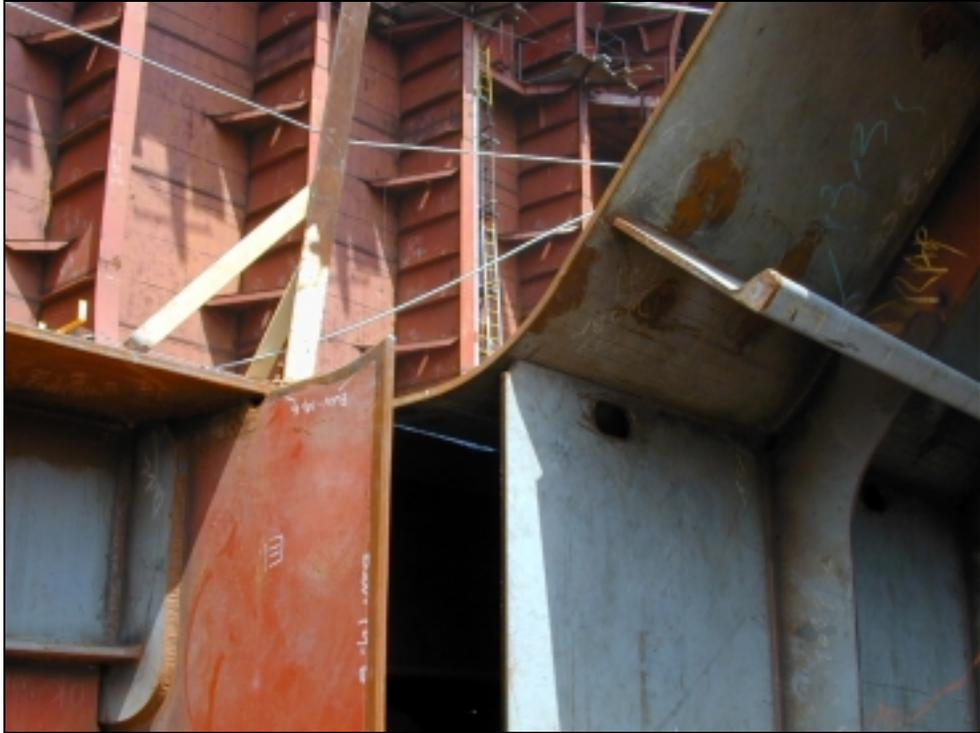
**Fig. A6** Detailed View of Hopper Connection, Looking from Below with Forward Unit Removed
