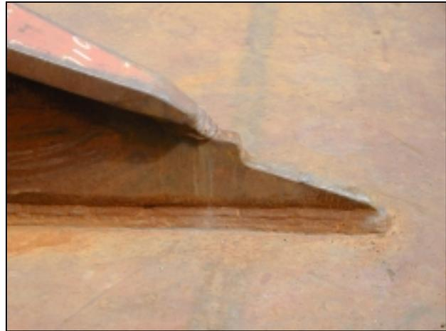
**Fig. A2** Detail of Transverse Web Frame Toe Attachment to Tank Top
