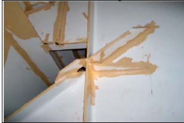
Figure 8. Structural Reinforcement – Bilge Bracket
